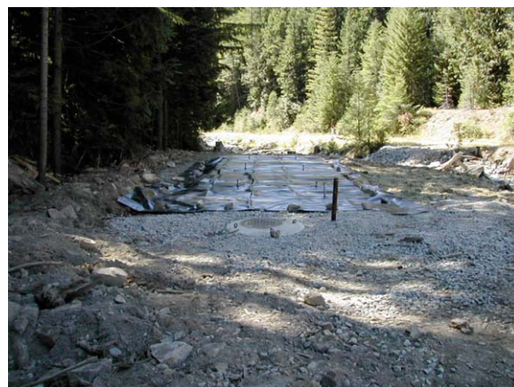
Fig. 4. The emplaced Apatite II PRB at the Success mine, between the East Fork of Ninemile Creek and the tailings pile, September 2002.
